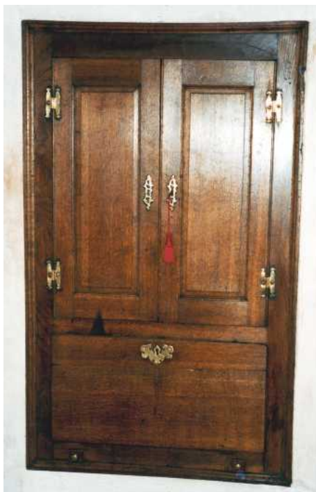
▲ Stripping and cleaning on site can be messy but is far easier than cabinet work and structural repair
